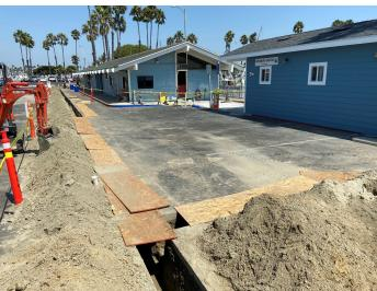
Electrical conduit trench from panels between restroom and fire station to edge of concrete walkway in front of NYCLB. Continuation will be from walkway thru grass area to new upgraded power panel in the NYCLB clubhouse. An additional line from the panel will then be routed to the new Shed building.
