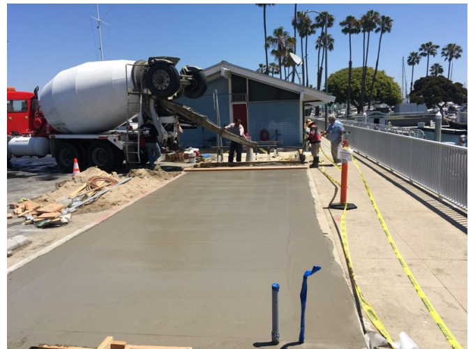
Pouring 11 cu. yards of concrete for the floor
