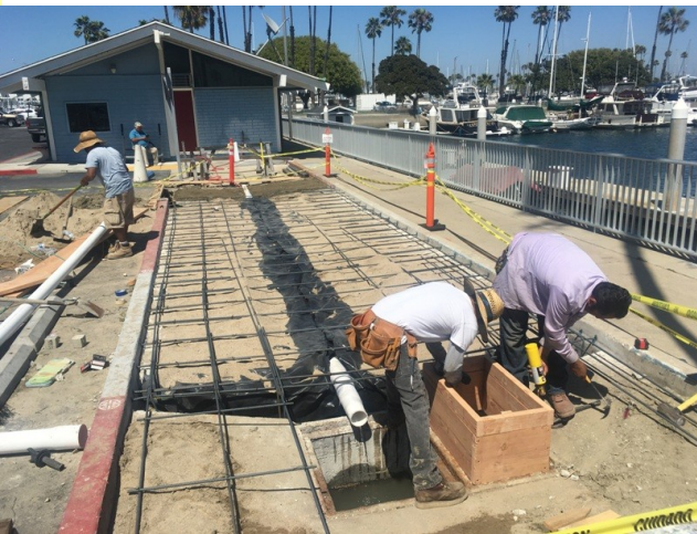
Locating the 4" drain line and setting rebar
