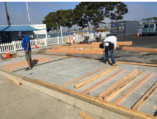
Laying out the first of the framing
